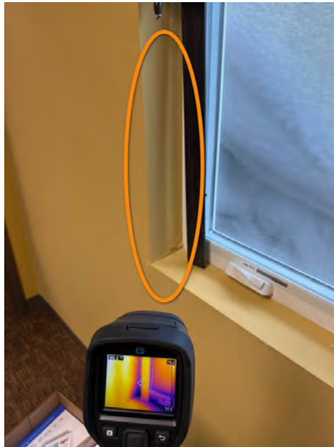
Northeast office closet
