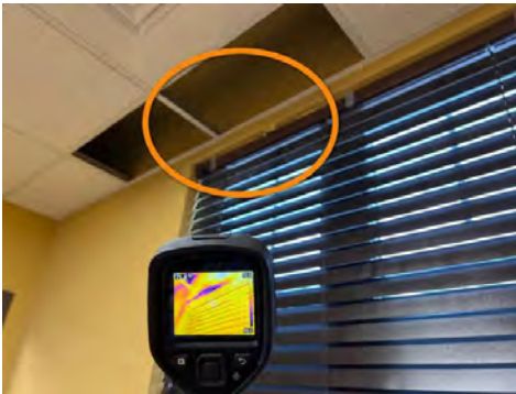
North east office closet
