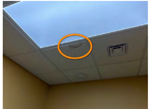
Northwest storage room
