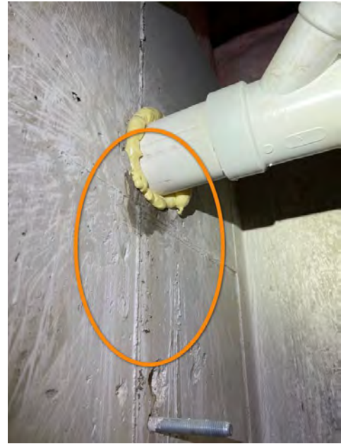
South Basement wall
