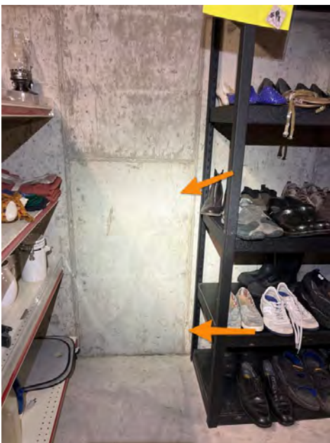
Northwest basement wall
