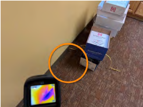
North east office closet
