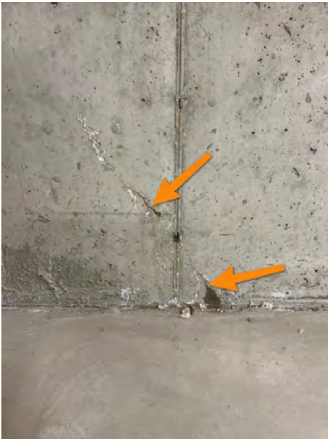
Basement Southeast wall
