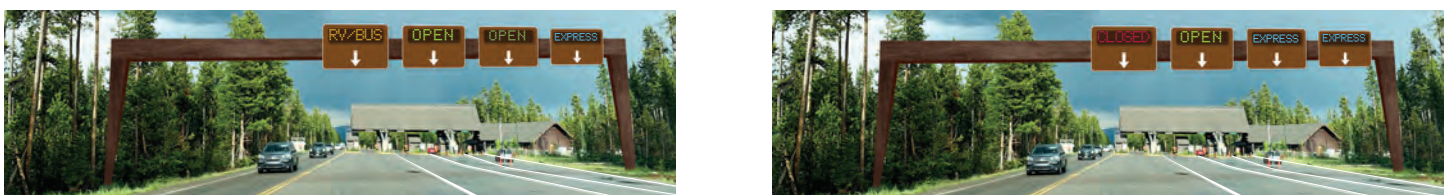
Figure 29: Proposed overhead gantry with “flexible lanes” signs that can be changed depending on current traffic needs.
