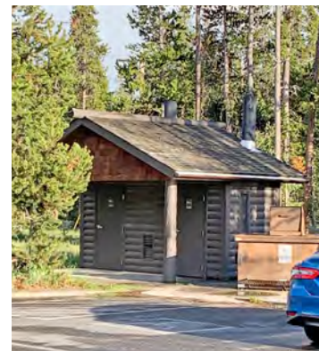
Figure 31: Current Restroom facility
