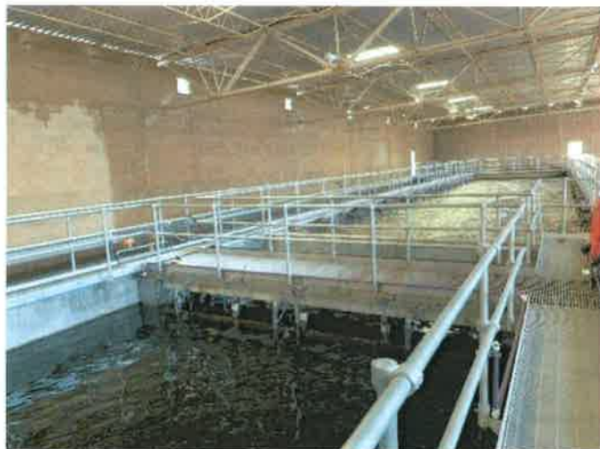
Figure I-8: Extended Aeration Process (Aero-mod)
