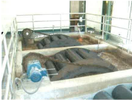
Figure I-10: IFAS Process (STM-Aerotor)
