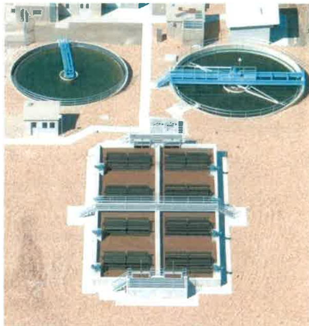
Figure I-11: IFAS Process (STM-Aerotor)
