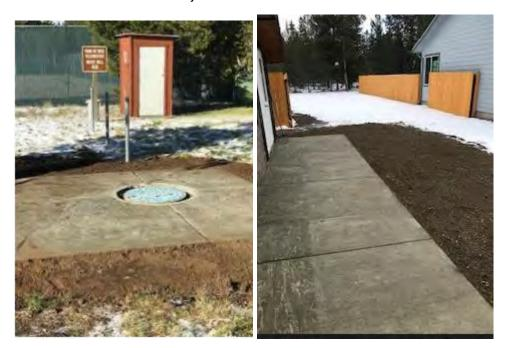
11-3-22: Preformed Water/Wastewater rounds. Collected wastewater influent/ effluent samples and sent to IAS Labs. Removed concrete forms form Madison station/Well #2 and injection well, back filled around the new concreate and made look nice.
