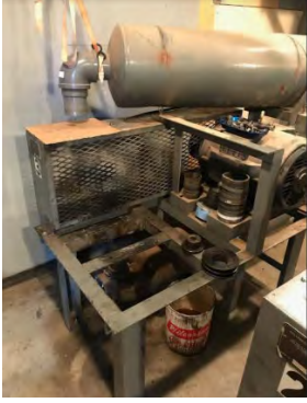
Removal of #3 blower
